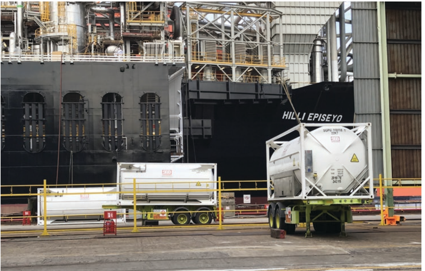
Regasification, LNG Transferring Service, and Provision of Equipment - The 1st commercial LNG bunkering project in Singapore
