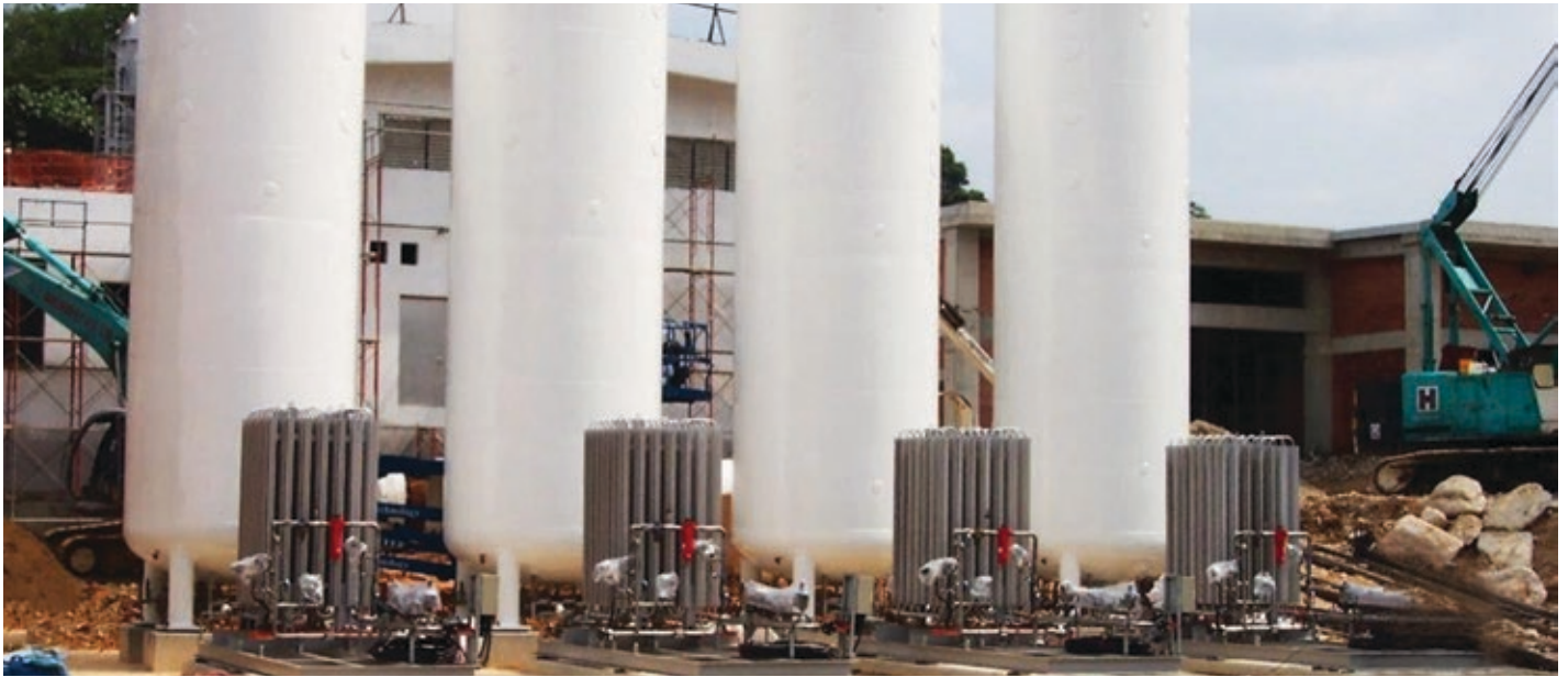
Provisioning and commissioning of storage and vaporization systems
